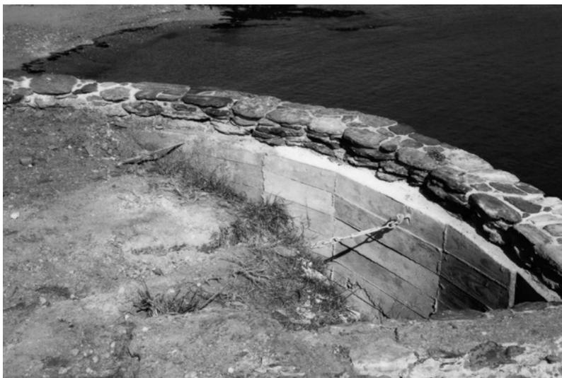
The project was started in the summer of 2009. Work proceeded to gradually pull the wall back without undo cracking. As sections of the wall became vertical, a concrete reinforcing wall was poured inside the wall to give it even more strength and wicks were installed throughout from inside to outside the wall to drain off any water that might collect.
